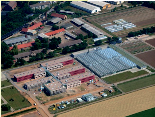
New BAZ complex on the Moorberg site
